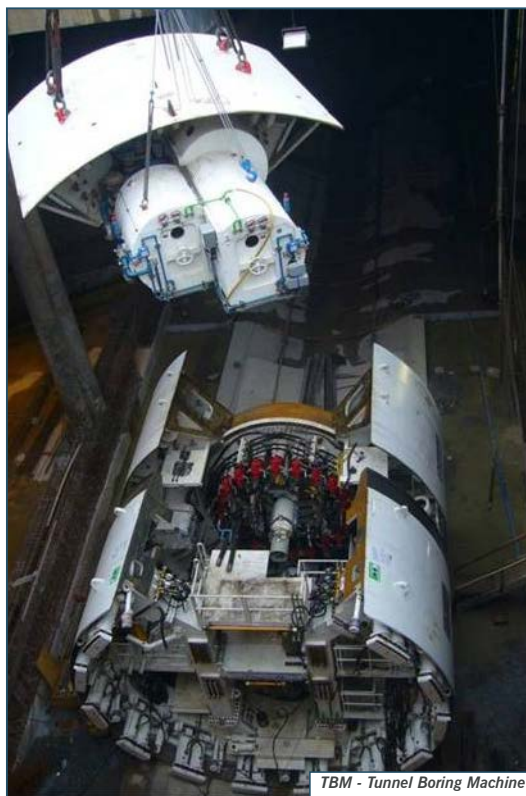
TBM - Tunnel Boring Machine
