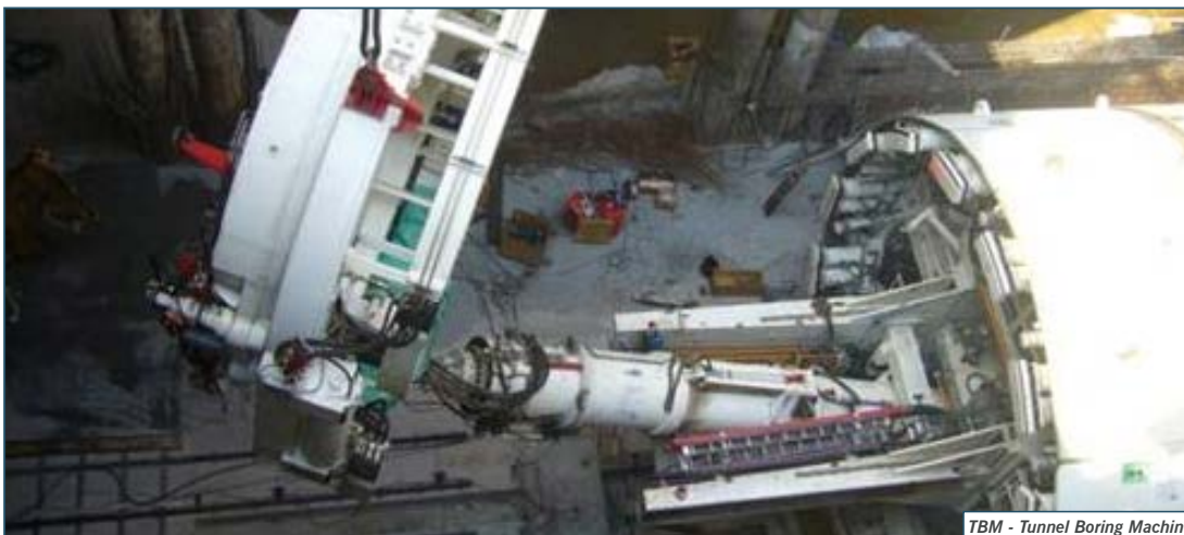
TBM - Tunnel Boring Machine
